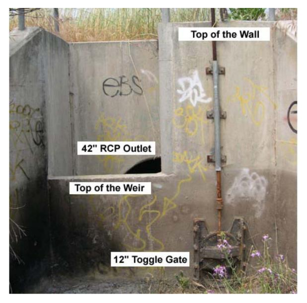
Figure 9 Photograph of Existing Marsh Outlet Structure
