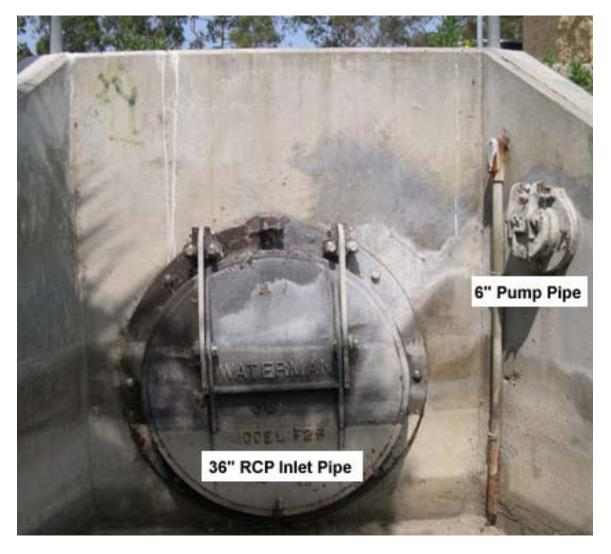
Figure 7 Photograph of Existing Marsh Inlet Structure
