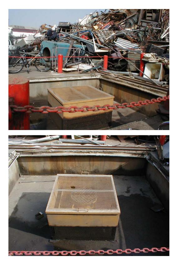
Figure 10. L.A. metal recycling yard BMP. Water flows through the grating of the metal top hat, into an infiltration trench.
